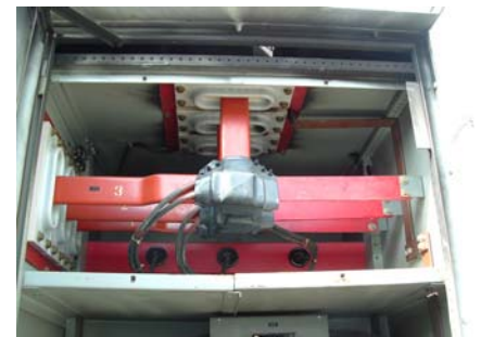
Re-designed, manufactured, repaired and installed
